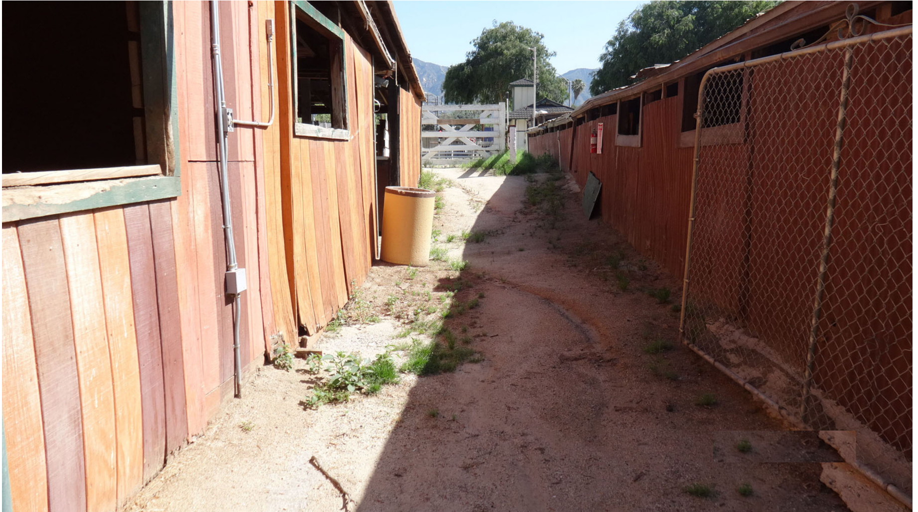
D. SOUTH-WEST CORNER BARN - EXTERIOR WOOD SIDING WALL DAMAGE ALONG WALL GRADE TRANSITION
