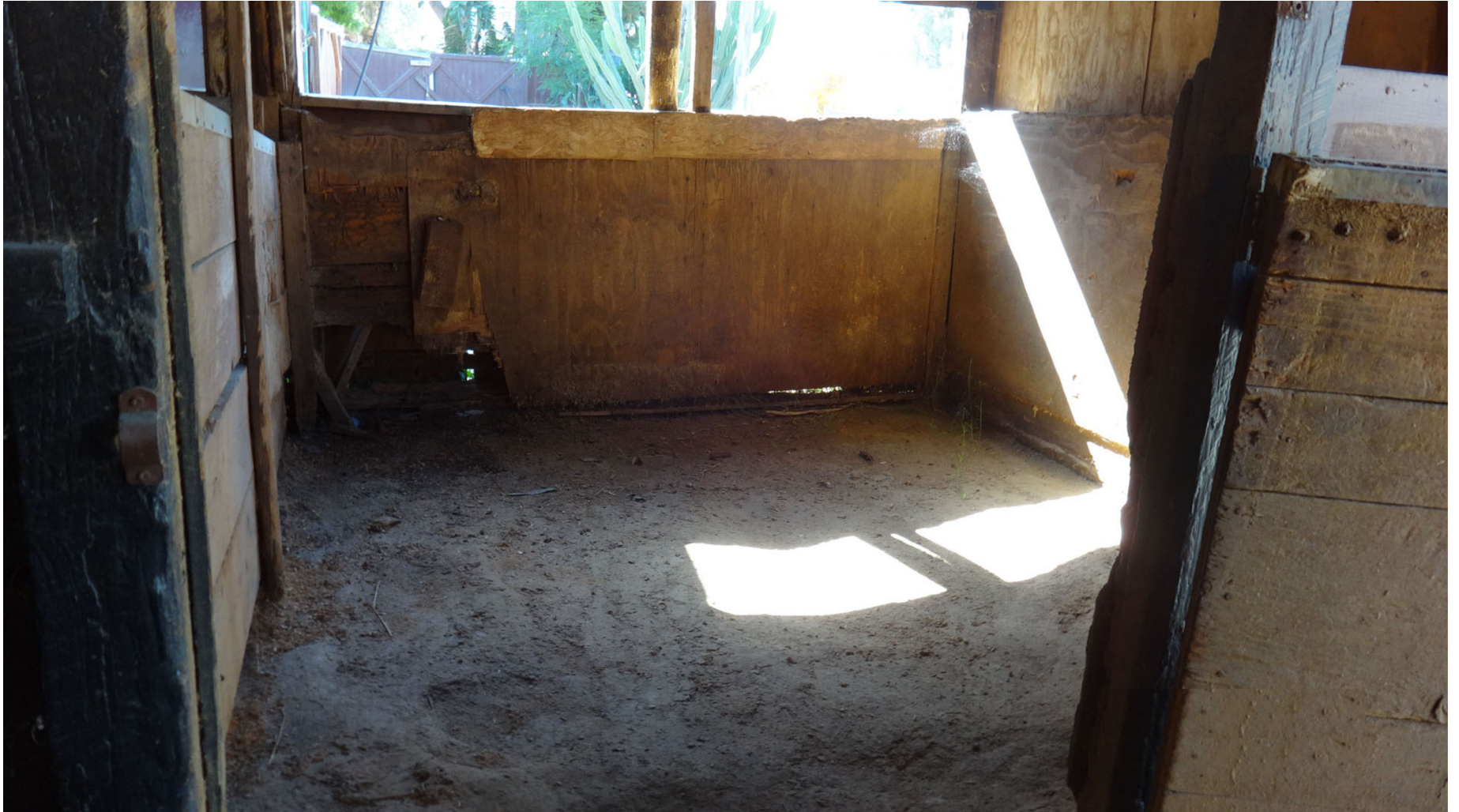
E. SOUTH-EAST CORNER BARN - EXTERIOR WALL CORRAL WOOD SIDING DAMAGE AND EARTHERN FLOOR DEPRESSION
