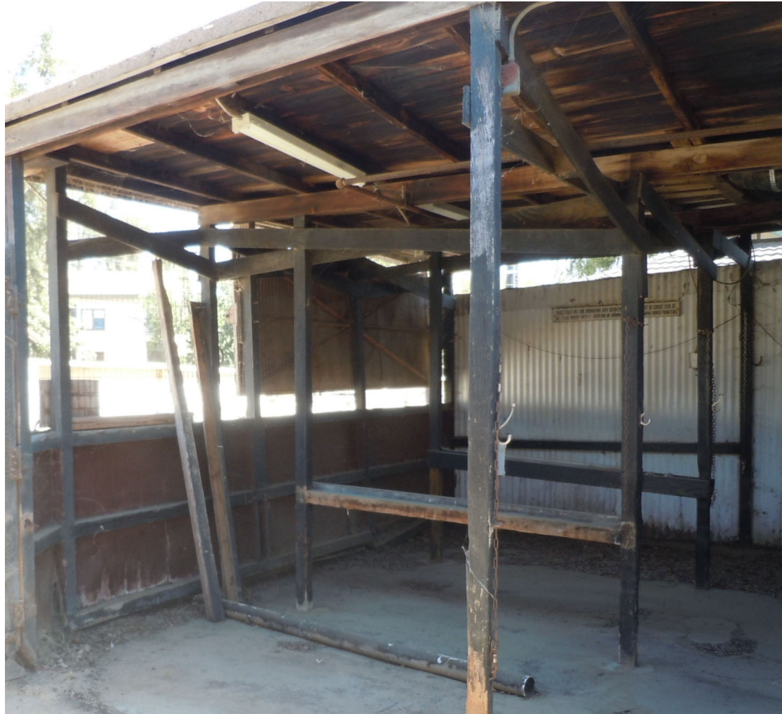
L. WEST BARN - EXISTING TACK, BRIDLE AREA AREA WITH METAL ROOF FRAMING DETERIORATED
