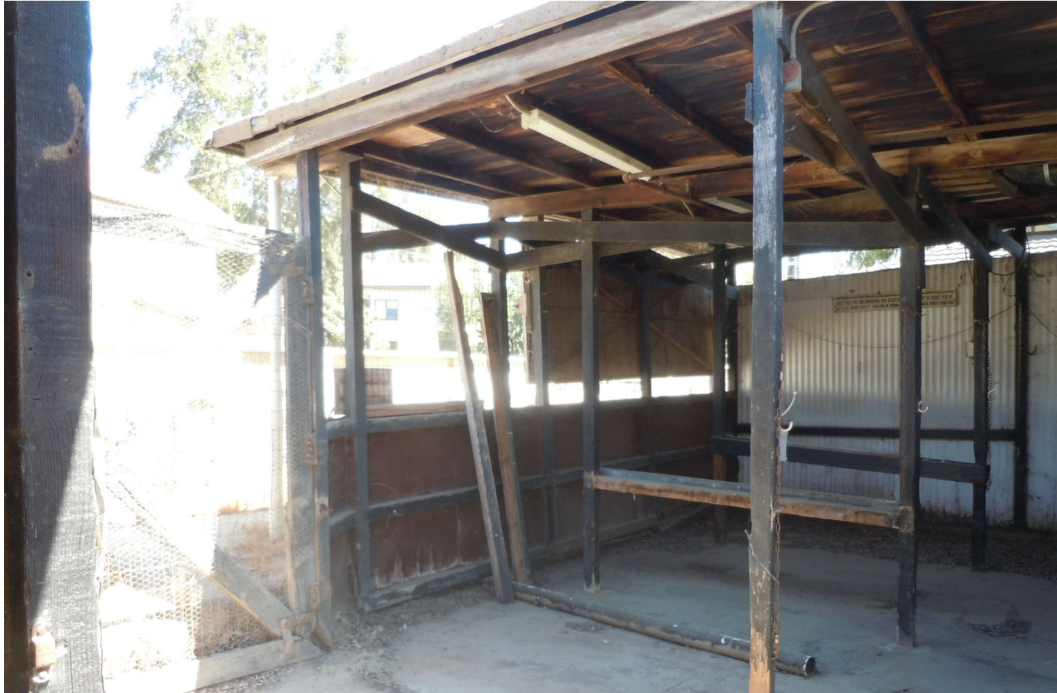
K. WEST BARN - EXTERIOR "V" METAL ROOF FRAMING AND TACK BRIDLE AREA DETERIORATED
