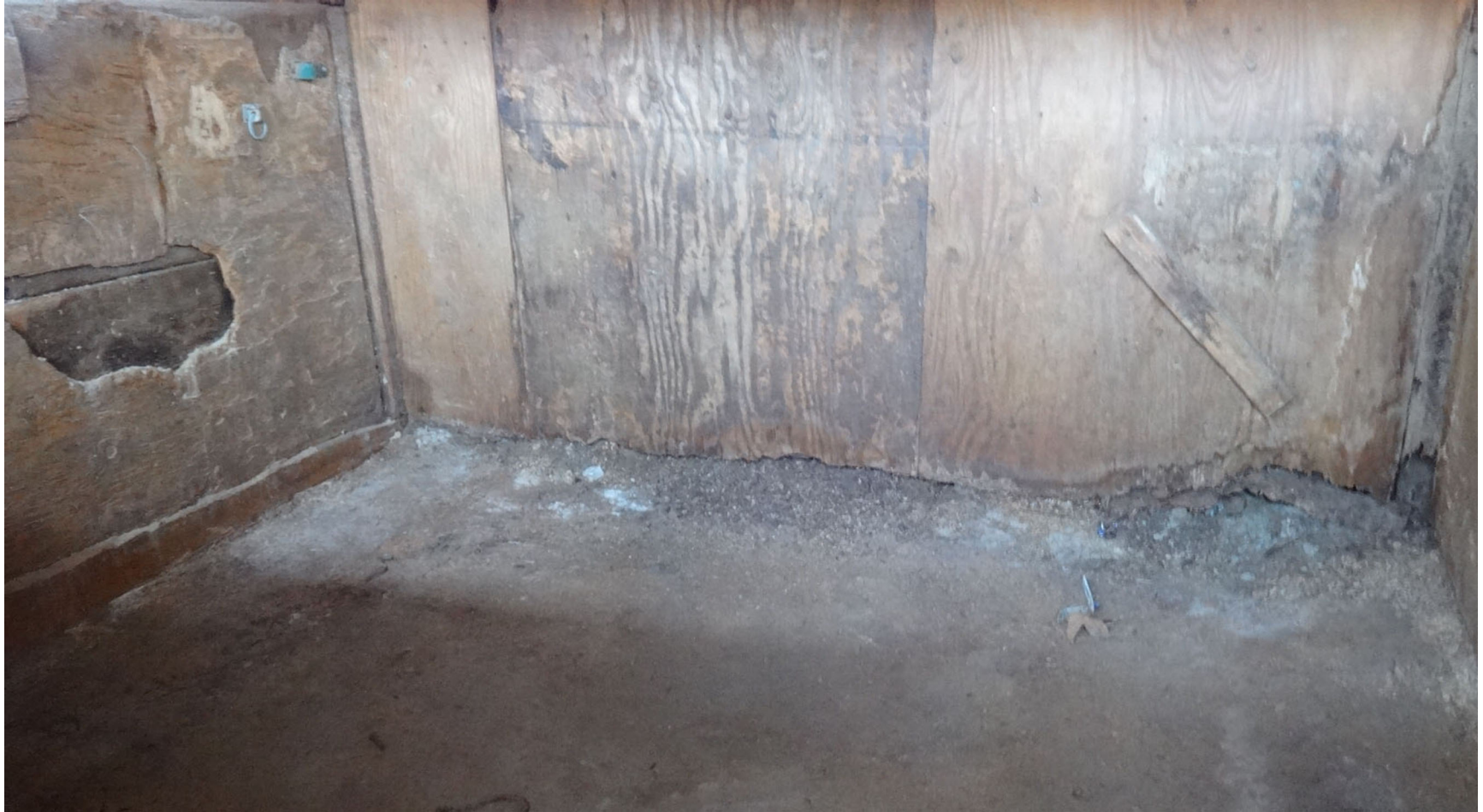
M. EAST STABLE - TYPICAL STALL WITH WOOD WALL DAMAGE. WOOD DAMAGE ALONG TRANSITION WITH EARTHEN FLOOR
