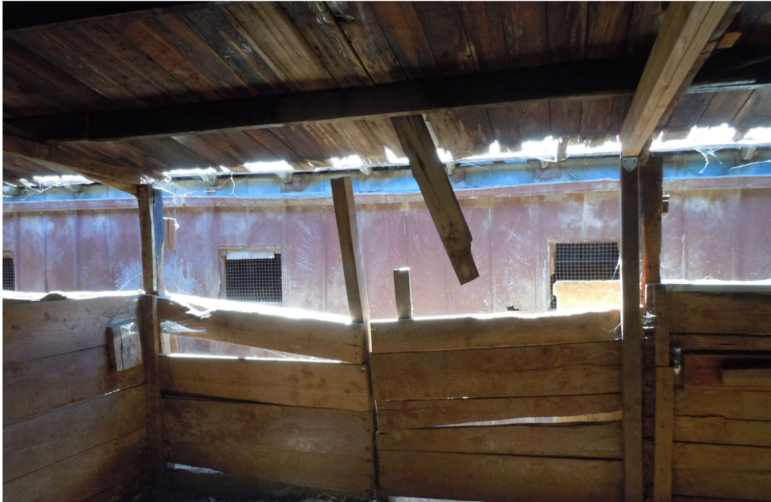
I. SOUTH BARN - EXTERIOR WALL WOOD CORRAL DAMAGED AND WOOD SHEATHING ROOFLINE EDGE DAMAGED.
