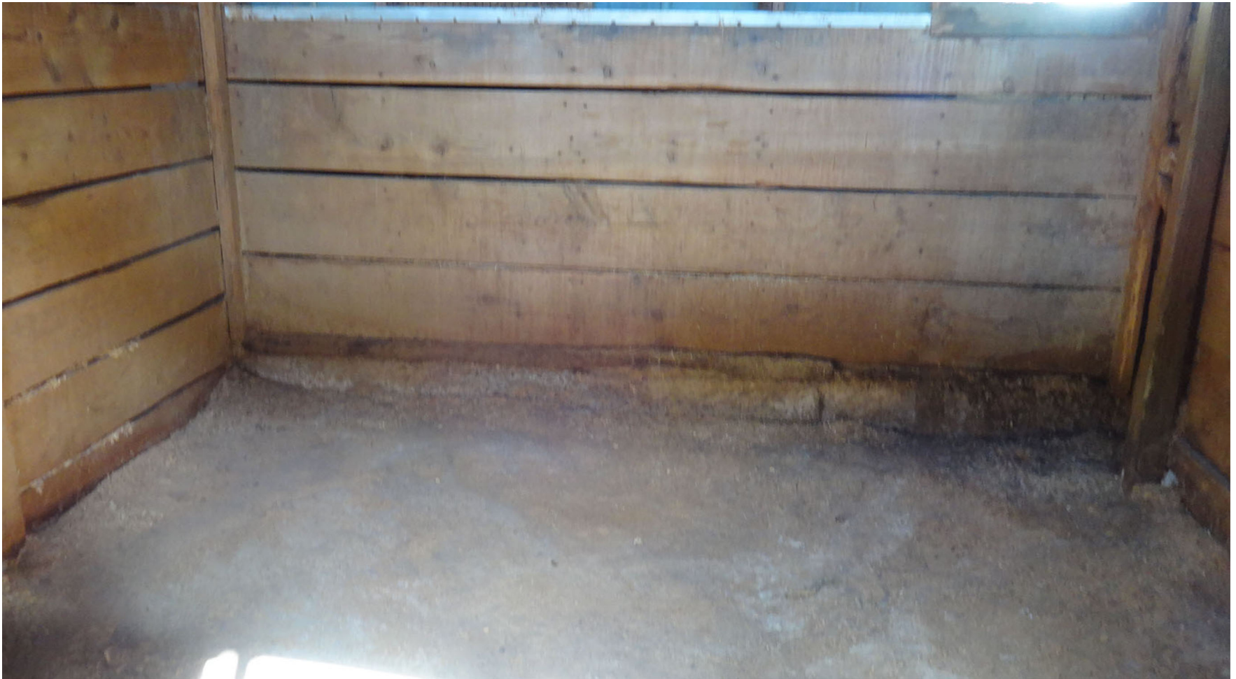
N. EAST STABLE - TYPICAL STALL WITH WOOD WALL DAMAGE ALONG TRANSITION TO EARTHEN GRADE. WORN OUT DEPRESSED PIT 8" TO 10" DEEP
