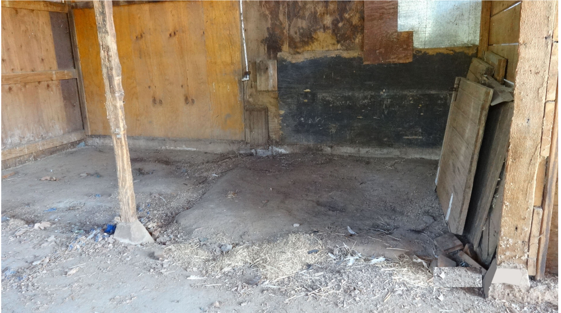
C. SOUTH-WEST CORNER BARN - EXTERIOR WOOD SIDING WALL PATCHED DAMAGE AND ROOF SUPPORT WOOD POST DAMAGE
