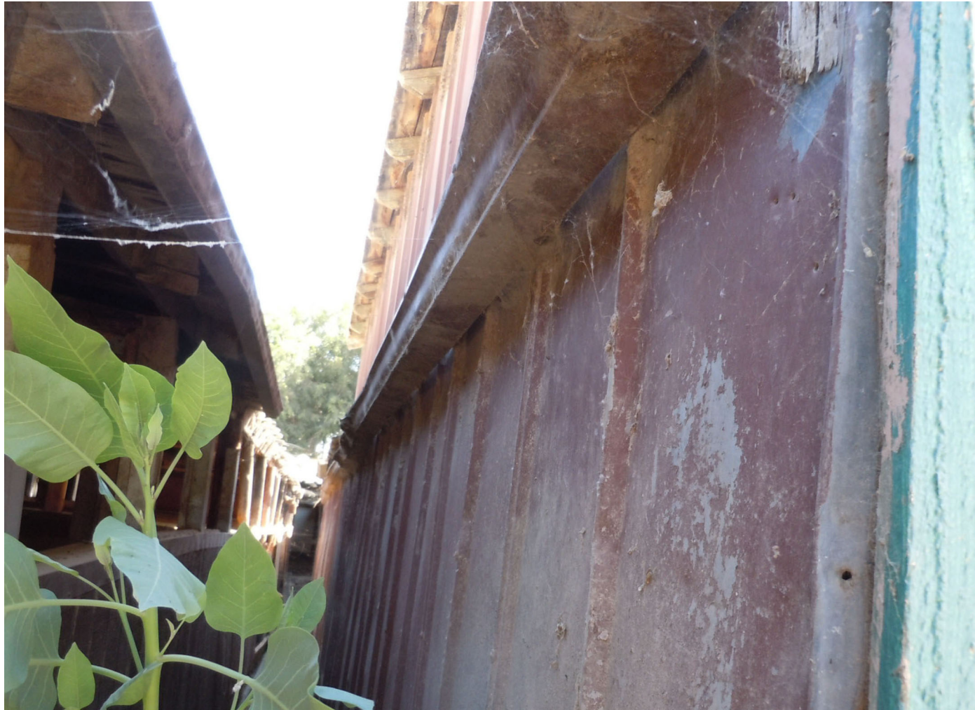
H. SOUTH-BETWEEN BARNs - METAL "VW" ROLLED WALL SIDING RUSTED CORROSION ALONG TRANSITION WITH EARTHEN GRADE. UPPER EXPOSED ROOF RAFTERS W/ WATER DAMAGED.
