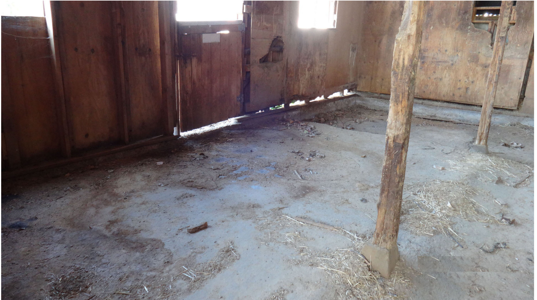
A. SOUTH-WEST CORNER BARN - EXTERIOR WALL WOOD SIDING DAMAGE ALONG FLOOR
