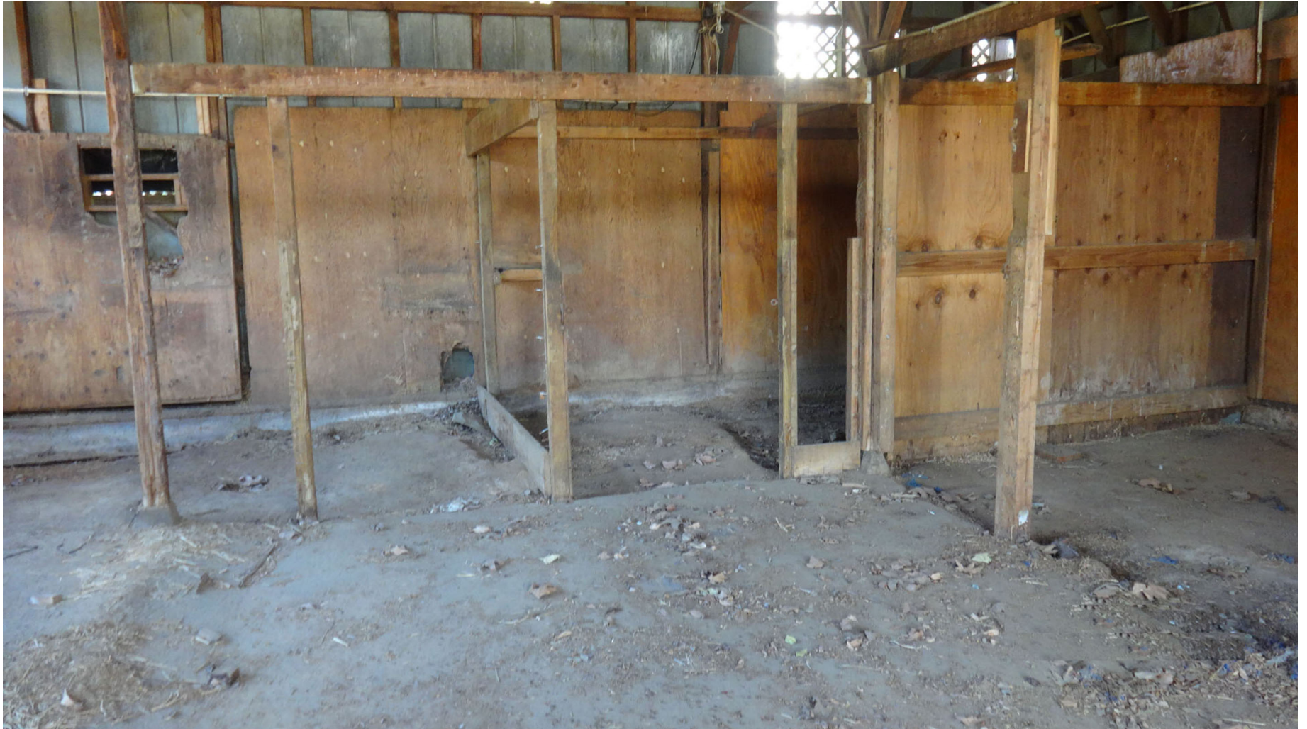
B. SOUTH-WEST CORNER BARN - EXTERIOR WOOD SHEATING DAMAGE AND ROOF SUPPORT WOOD POSTS DAMAGE
