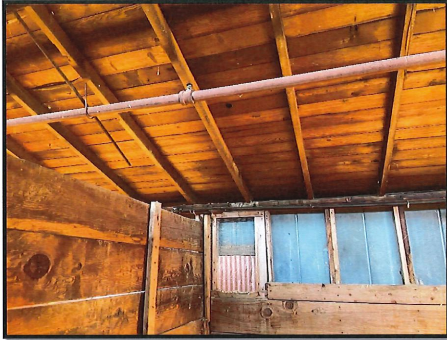
Photo #5 Typical Longitudinal wall at Eastside Stable
