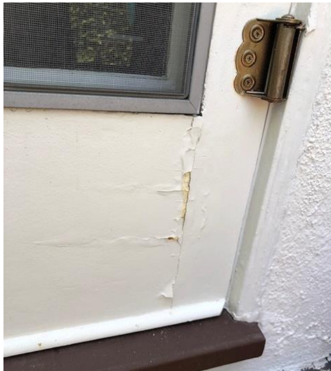
15. 2795 Mira Vista Drive, Door Jamb Separation Detail, June 2022
