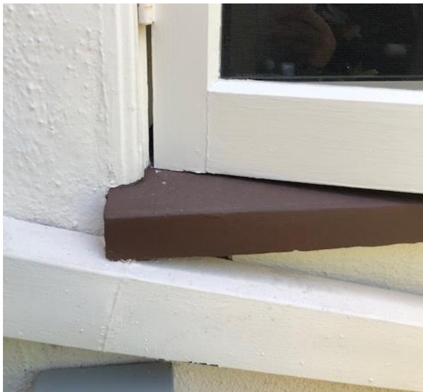
17. 2795 Mira Vista Drive, Window Jamb Separation Detail, June 2022
