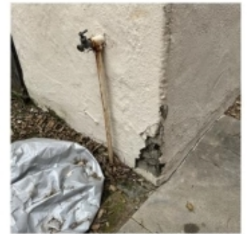
Localized spalling at painted stucco facades.
