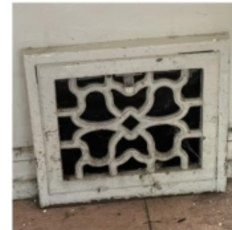
Original cast iron vent covers to be restored and possibly reused.
