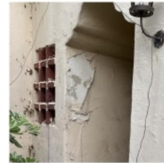
Hairline cracks and peeling paints at painted stucco facades.
