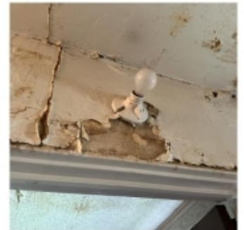
Water damage at ceilings and walls.
