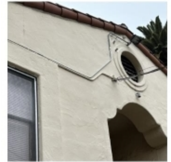
Misc conduit & wiring mounted across facade, connected to contemporary light fixtures.
