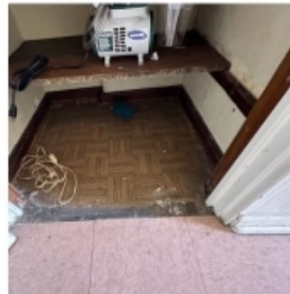
Multiple layers of vinyl flooring throughout; requires asbestos abatement.
