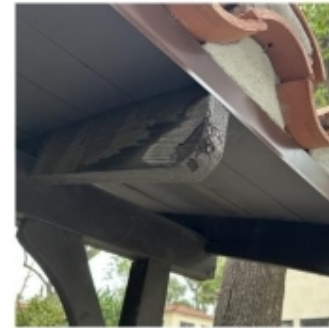
Peeling paint and splitting at wood posts, joists, and beams.
